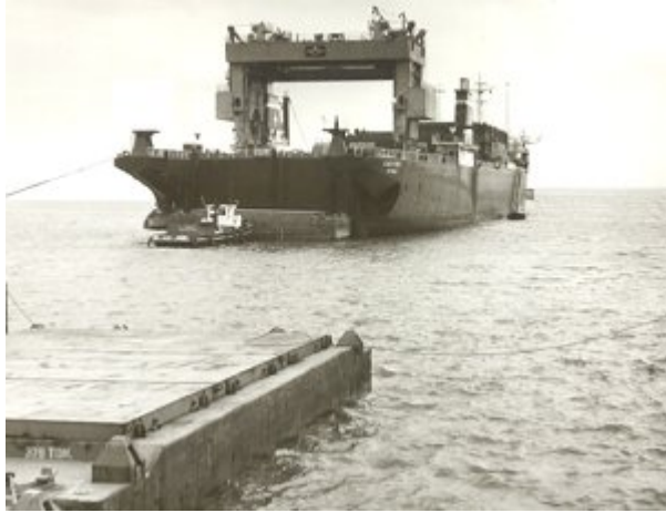
Embarking LASH barges in the floating area
