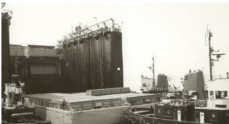
Floating a barge over the lowered winch platform
